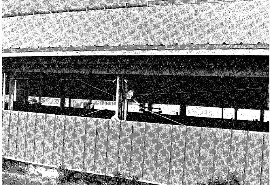
*Adjustable panels and openings under the eaves are incorporated in this naturally ventilated building.*
